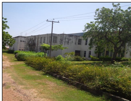
Fig 3: Access Road to the Library Complex with Grasses Growing on it (Source: Authors' Field Work, 2018).
