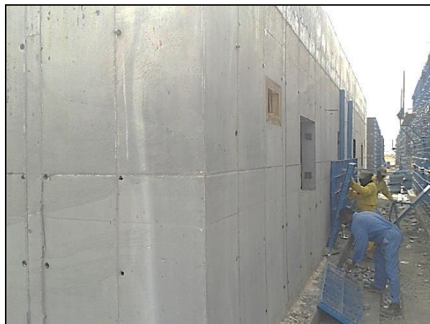
Fig 5: Open the Molds after (20 days)
