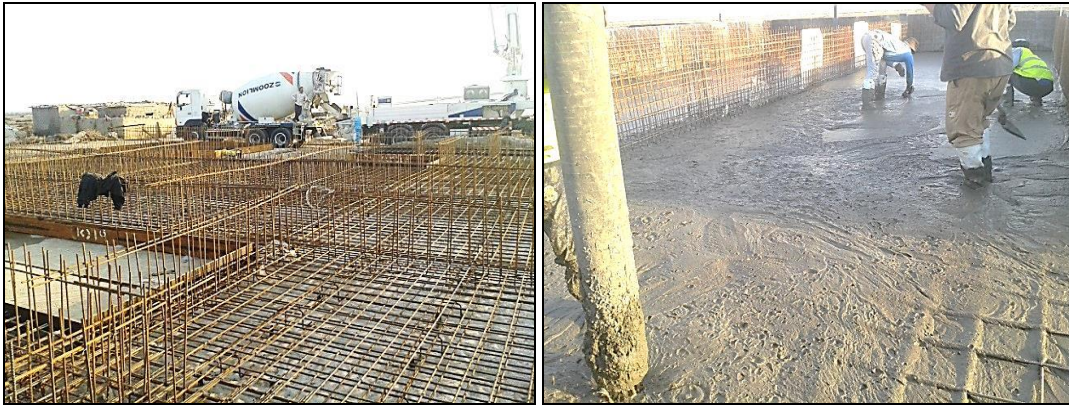
Fig 2: Details of steel reinforcement and casted the foundation
