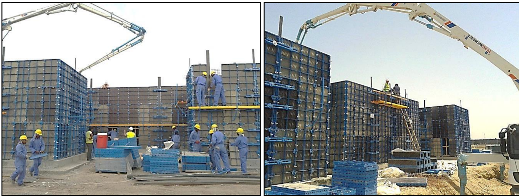
Fig 3: Put the Molds before the casting
