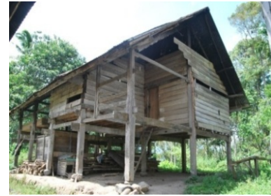
Photo 3: Umah Belah Space
