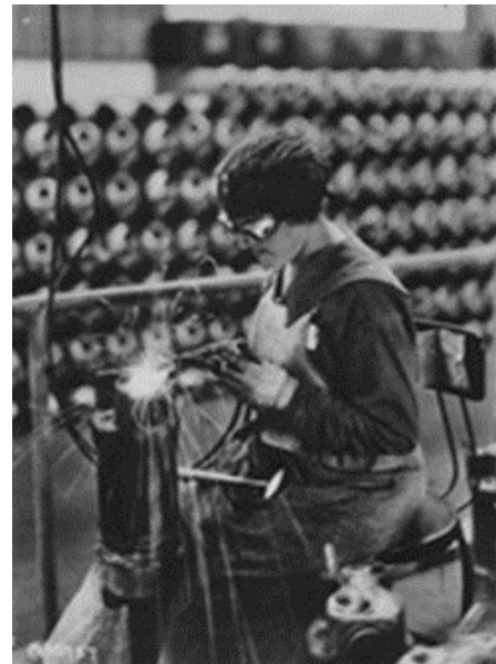
Acetylene welding on cylinder water jacket, 1918
